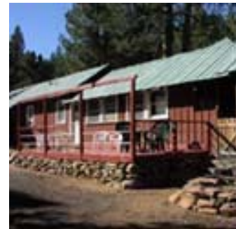
Figure 6. Laboratory building at Sagehen Creek
